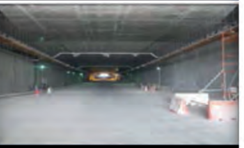
NDIA Tunnel – (Doha, Qatar)
